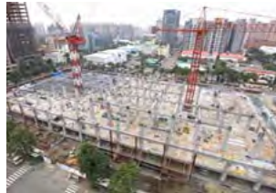
pre-cast Base construction
