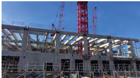
Pre-cast exterior wall panels are constructed without outer frames
