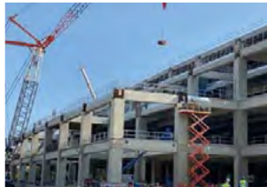
Pre-cast exterior wall panels are constructed without outer frames
